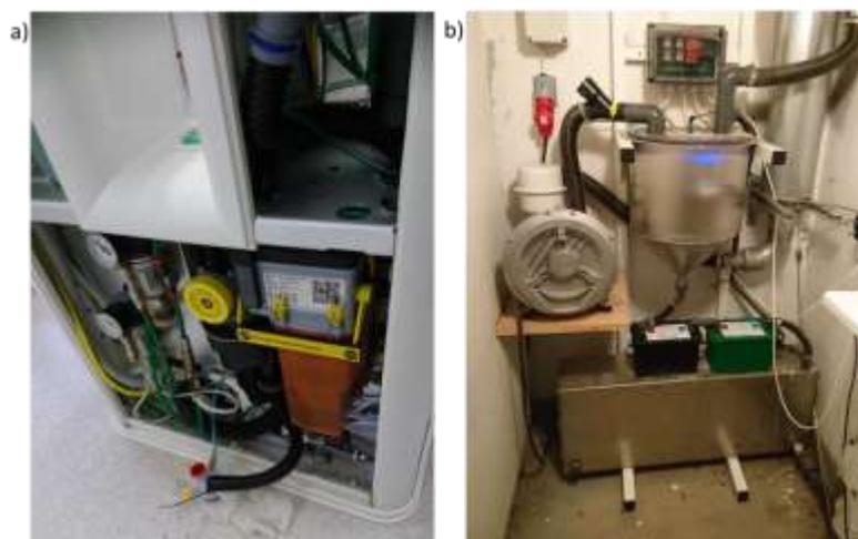
**Figure 3** a) Water sampling point after an amalgam separator installed in a chair unit, b) Water sampling point after amalgam separators installed at the water outlet of a clinic.
