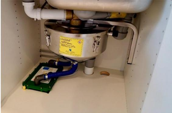
*Sink amalgam separator with surge tank, installed beneath sink.*
